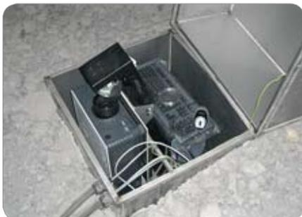
Due to "aggressive" salty dust the technical equipment has to be covered and cooled properly
